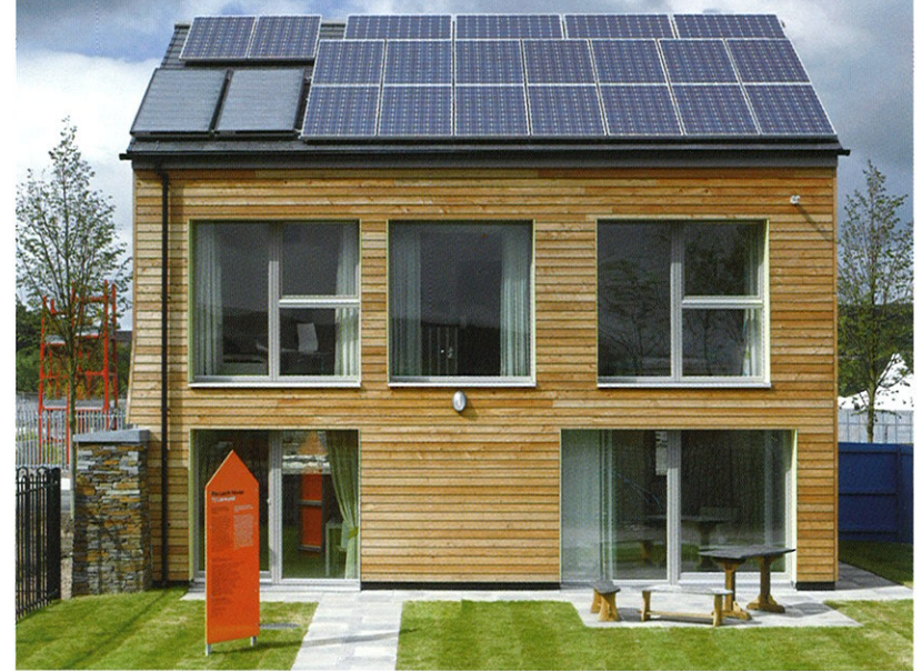
THE LARCH HOUSE The UK's first zero carbon (code 6), low cost, certified Passivhaus, built as prototype social housing utilising NBT systems and support, launched at this year's National Eisteddfod for Wales.
