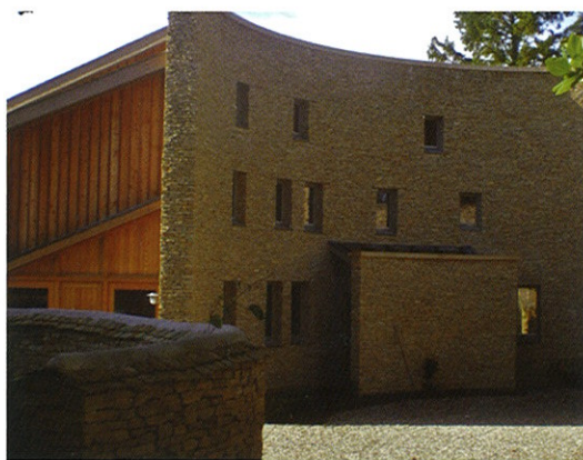
NBT's ThermoPlan structural insulation system enabled an architecturally striking 8.5m tall supporting wall to be built on a curve to form the north facing elevation of this private house development in Charlbury, near Oxford. The system delivers high levels of thermal and acoustic insulation and highly effective breathability, whilst also providing crucial thermal mass, which helps to prevent summertime overheating of the, otherwise, lightweight building.
