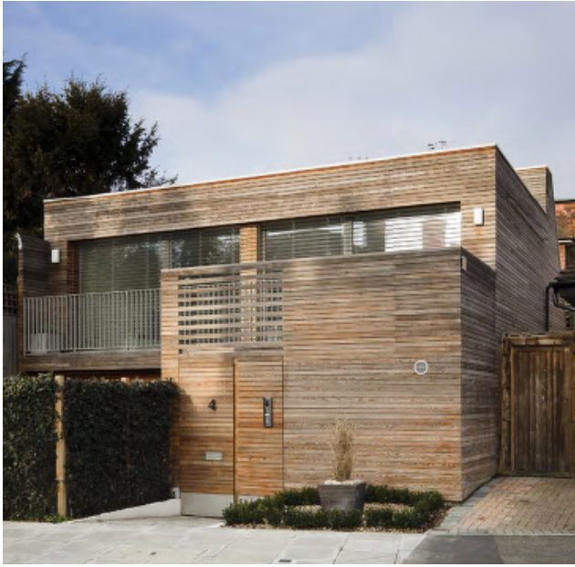
South and east facades of the house
