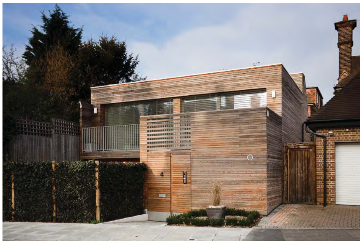
The house is a modern, timber-clad design with exceptionally low heat loss and excellent air tightness
