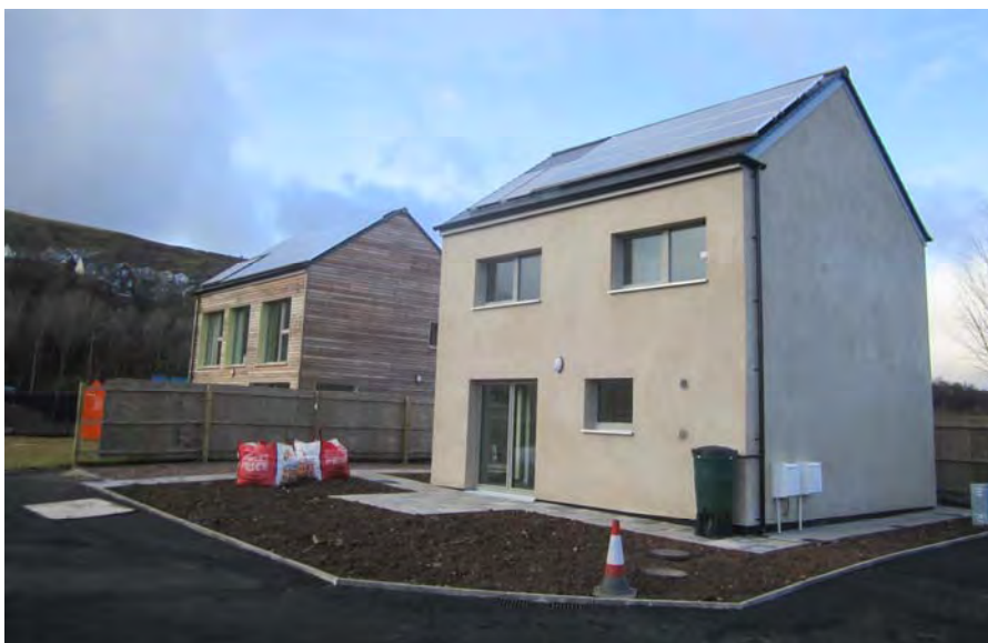
Figure 2-17. The Lime House nearing completion.
