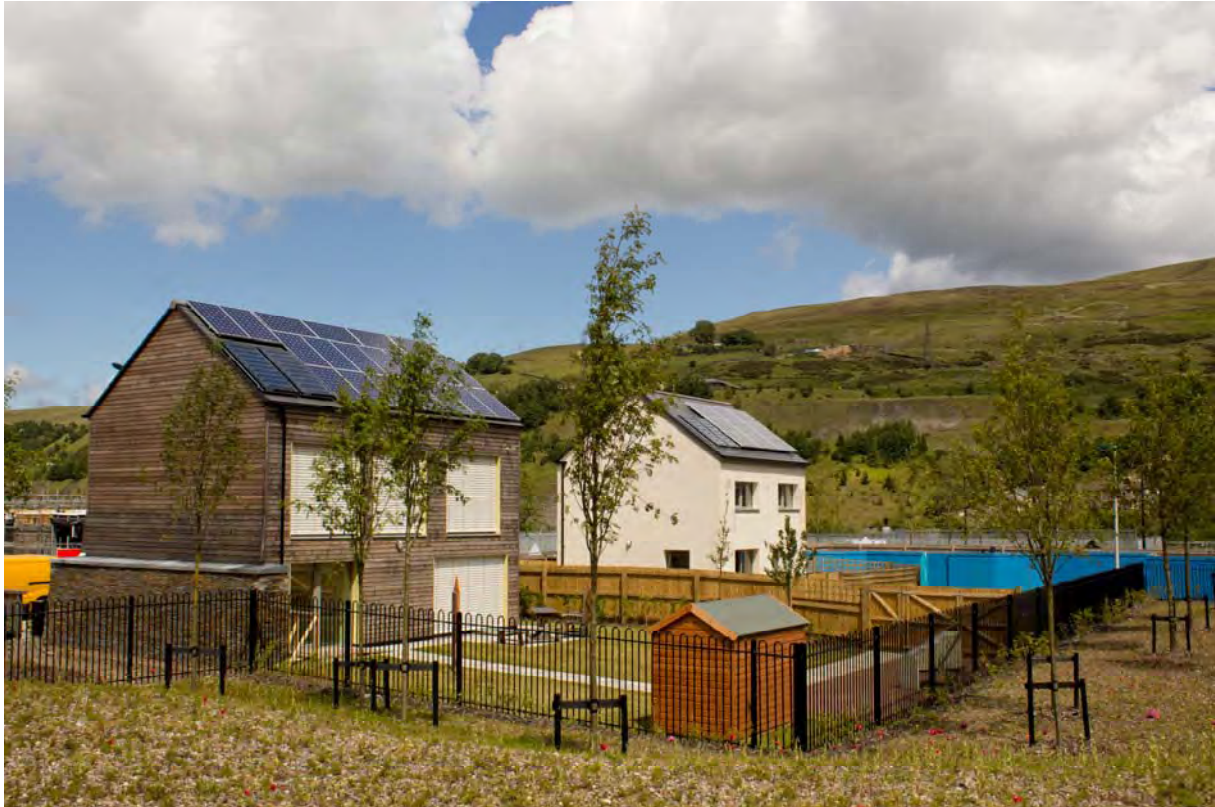
Figure 1-2. The Larch and Lime Passive Houses (backyard view)
