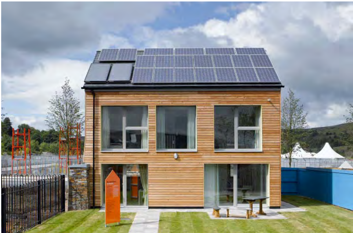
Figure 2-2. South facade of the Larch House with large windows and retractable external blinds.
