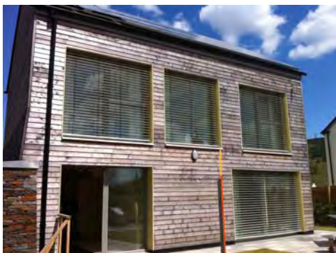
Figure 8-8. External blinds at the Larch House.
