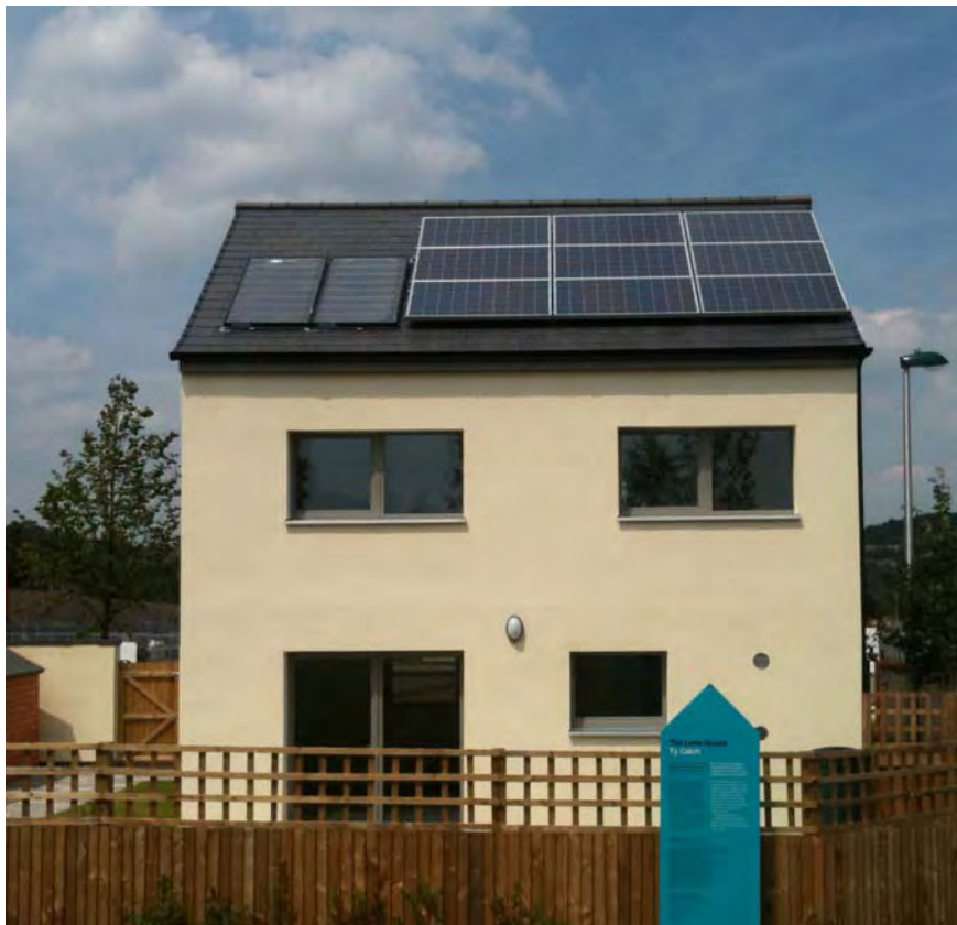
Figure 2-5. Lime House - south facade with smaller windows than Larch House.
