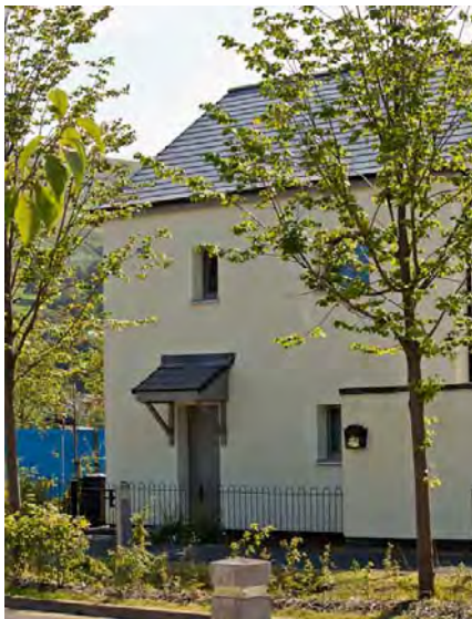
Figure 8-4. The Lime House front facade
