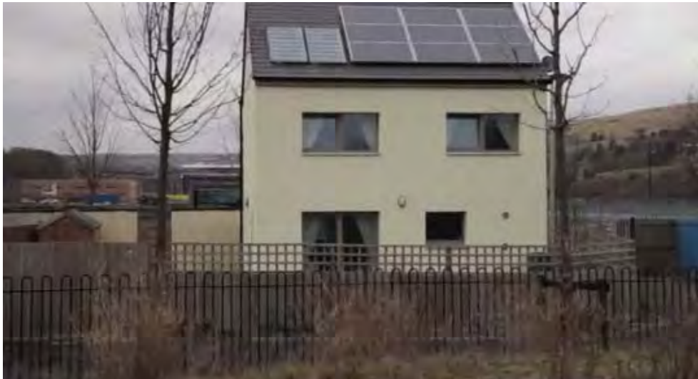
Figure 5-3. The Lime House showing the first floor bedroom and hallway windows tilted in the open position. Further investigation revealed that they were habitually left open almost constantly during the winter.
