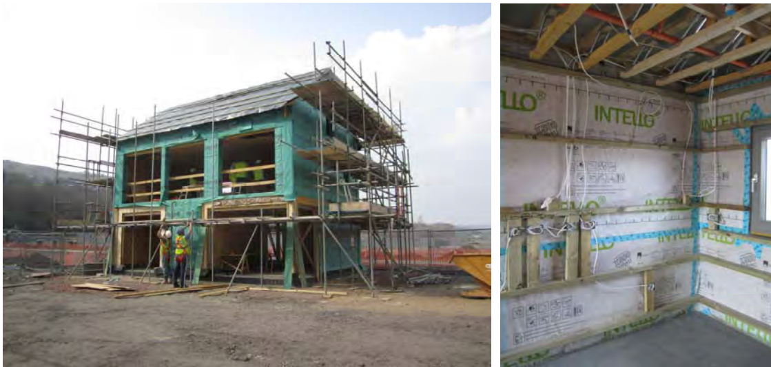
Figure 2-16. The Larch House under construction
