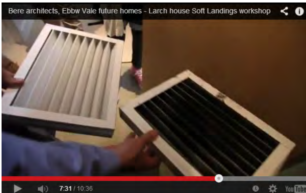
Figure 5-1. Still from the short film created from the summer workshop at the Larch House showing the difference between the clean and the dirty filters, July 2012 (authors bere:architects & Carmen Zografou)
