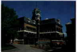
Abbey Mills Pumping Station © Thames Water
