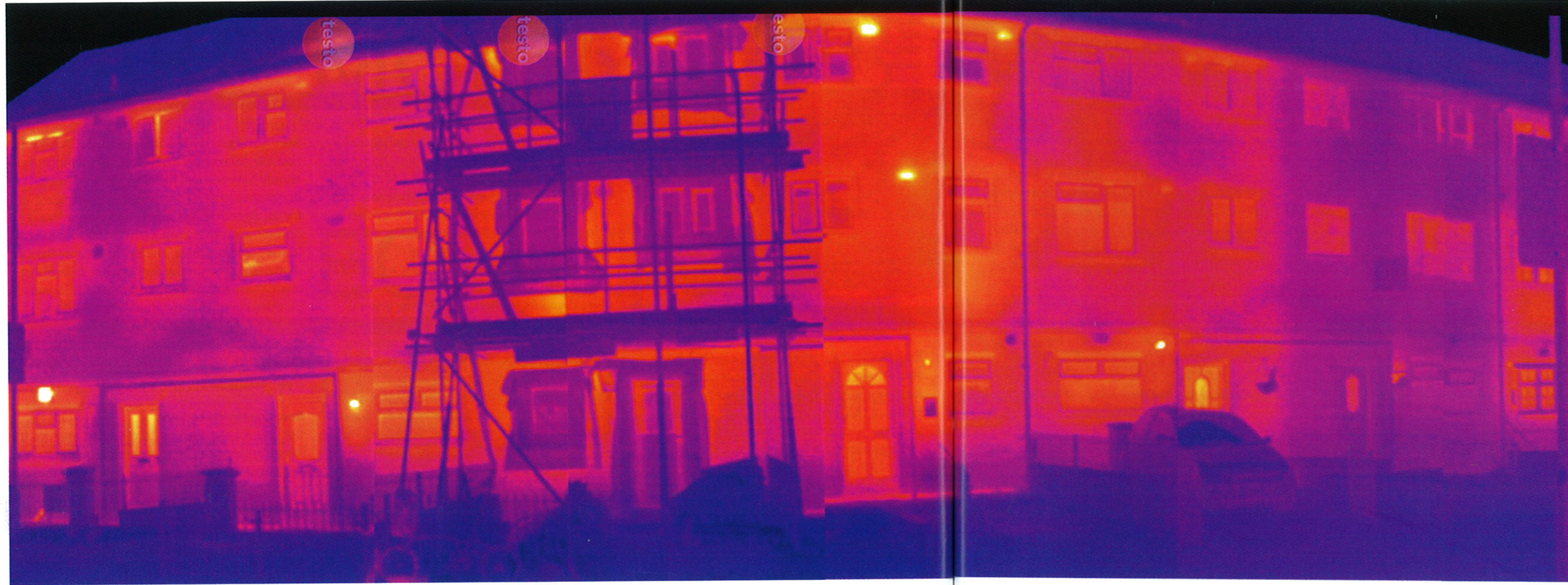
LEFT: Bere:Architects' thermal image shows their project behind scaffolding and the heat loss from single glazed windows to the left.
